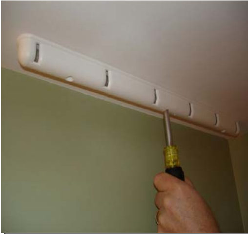
Console on the wall clasp side should be about 2”- 3” (5-8cm) from the wall. Attach consoles to the ceiling. Distance between centers of consoles: 42” (107cm).
