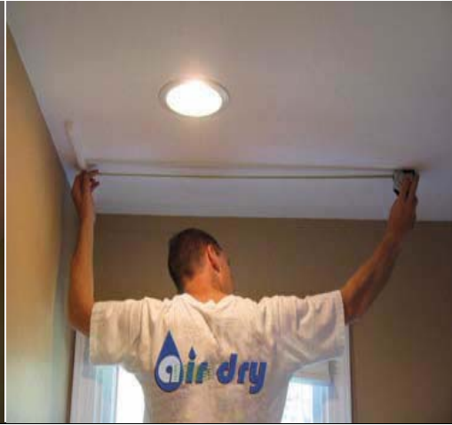
Console on the wall clasp side should be about 2”- 3” (5-8cm) from the wall. Attach consoles to the ceiling. Distance between centers of consoles: 42” (107cm).
