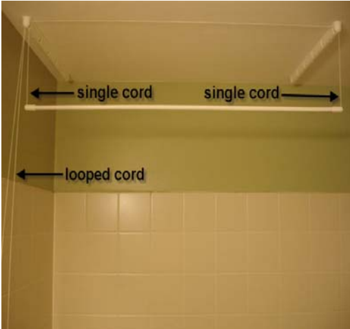
Pull cord through consoles as shown on the photo. (Use supplied bobby pin)
