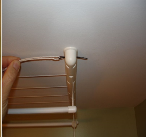
Pull cord through consoles as shown on the photo. (Use supplied bobby pin)
