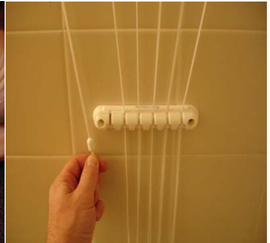
Tie a knot for bead 1 – so that the rod is in the ceiling position. Tie a knot for bead 2 – so that the rod is in a comfortable position for hanging wet clothes.
